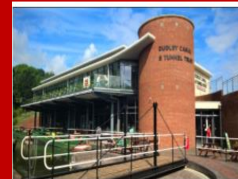
Dudley canal and tunnels
