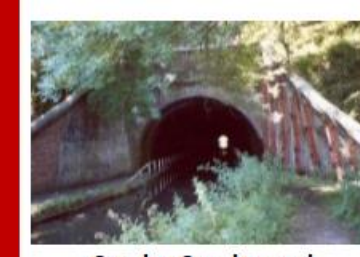
Coseley Canal tunnel
